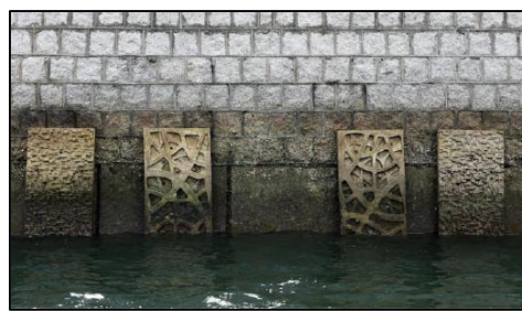
Use of locally-manufactured eco-materials at Pier Foundation
